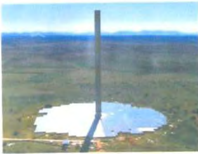
Prototype of the solar tower prototype plant at Manzanares, Spain
