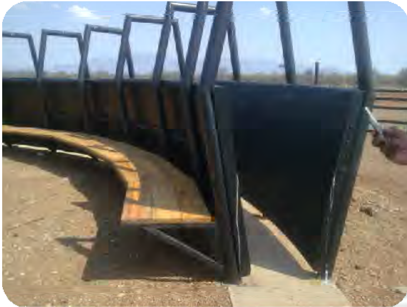
Constructed Box Shaped Crash Assembly
